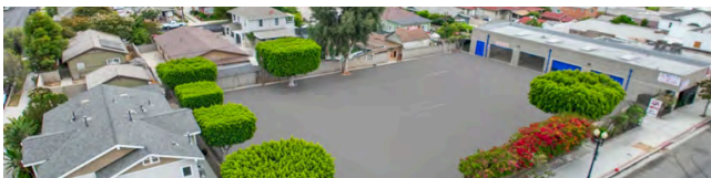
PERIMETER GATE & BLOCK WALL
